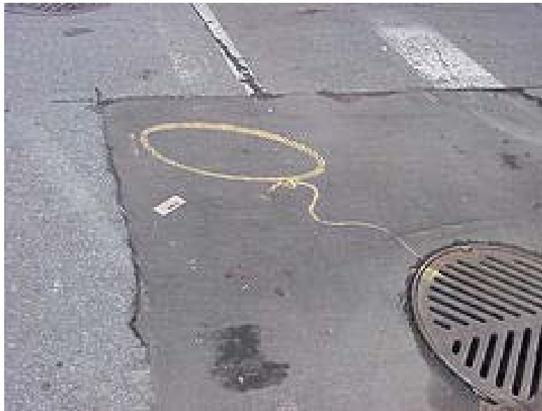
Fig. 3. Lasso tied to manhole cover.
